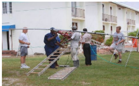
Initial assembly of the 6M7 Antenna
